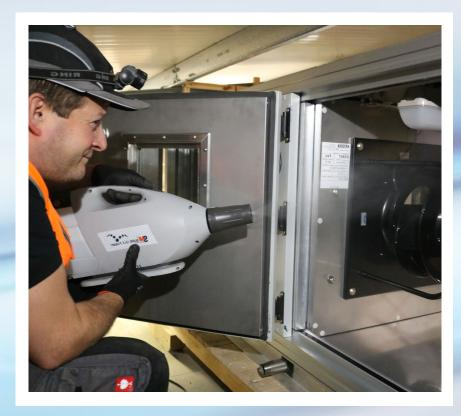
New H13 HEPA filtration was then installed. Following the installation of the new filters, the AHUs were fogged once again to eliminate any remaining bacteria and virus particles.
